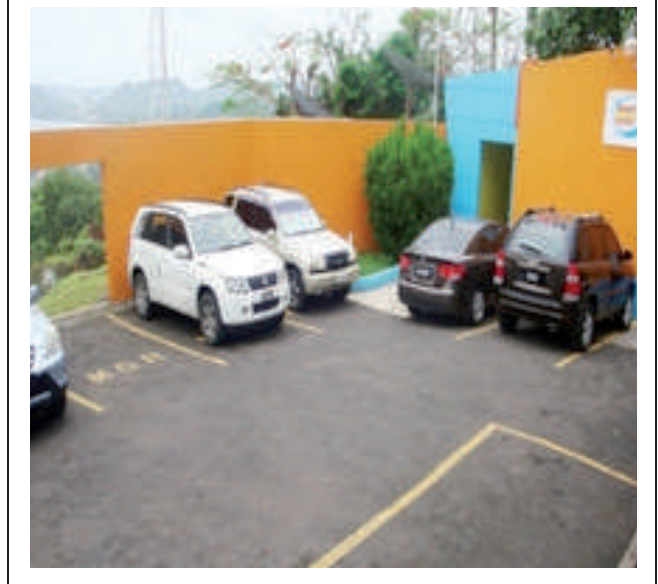
Radio Saint Lucia before and after renovation works
