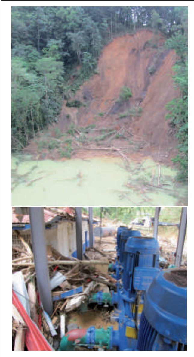
Damage suffered by the water sector after the December 24th Trough
