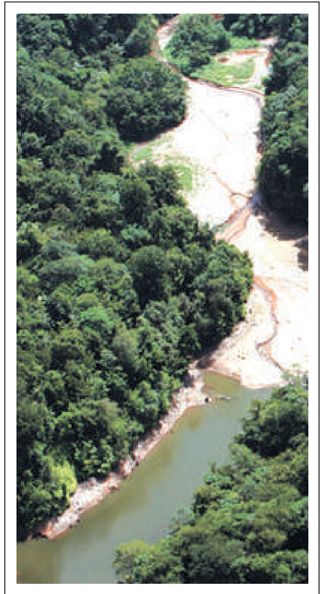
Heavy siltation at the John Compton Dam
